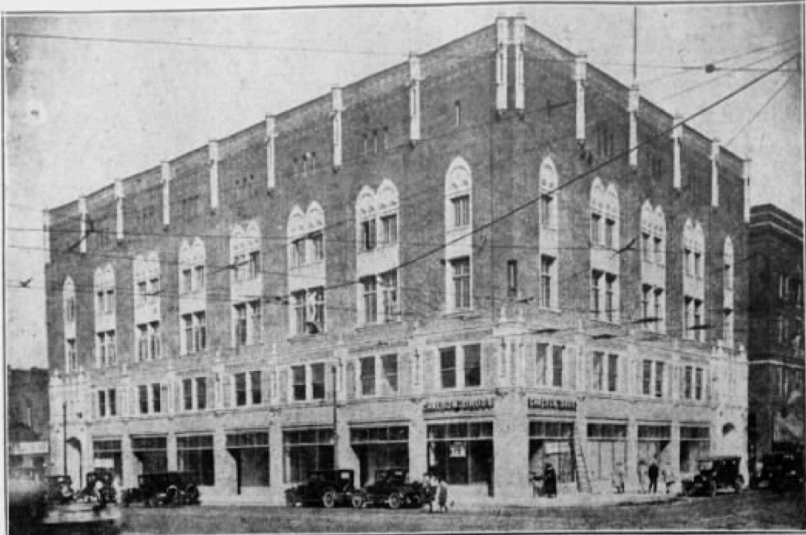
This new five-story building, nearing completion at Fourth street and Central avenue, has been erected by the Cataract lodge, No. 2, A. F. & A. M. at a cost of approximately $325,000. Contractors are now completing the interior and the structure will be ready for formal opening in about 60 days. J. A. Jensen, chairman of the building committee, said Saturday. The building was designed by Fallows & Huey, Minneapolis architects and the contractor is R. S. Billingsley.
